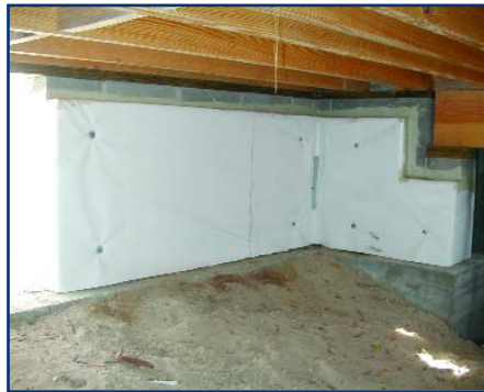
This crawl space under construction has careful detailing at all beam pockets to maintain the termite inspection gap at every interface of masonry and wood.
