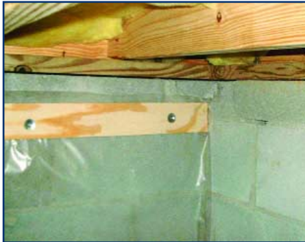
One way to mechanically attach a wall vapor retarder: secure it behind a preservative-treated plywood furring strip attached to the masonry with nails driven through washers. Photo credit: Bill Warren.
