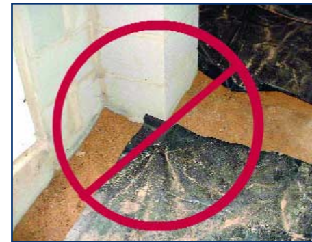
Do not leave any exposed earth in the crawl space! Photo credit: Bill Warren.
