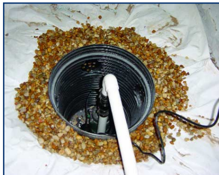
Use sump pumps if desired or when gravity drains are not feasible. This model includes a cap for the housing and an optional liquid water alarm to detect a failure of the sump pump system.
