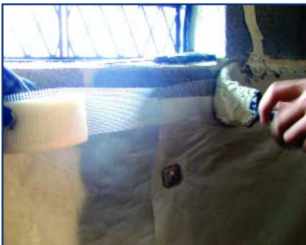
This heavy-duty vapor retarder material is mechanically supported by metal pins with cap washers and sealed to the masonry with fiberglass mesh tape and duct mastic. Photo credit: Indoor Environmental Systems.
